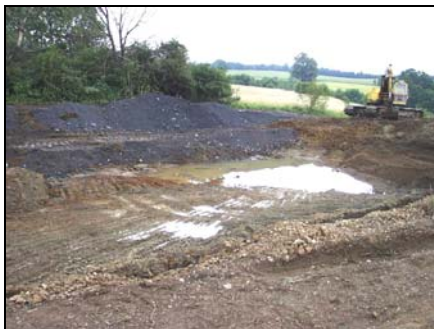
Removing sludge from the lagoon
