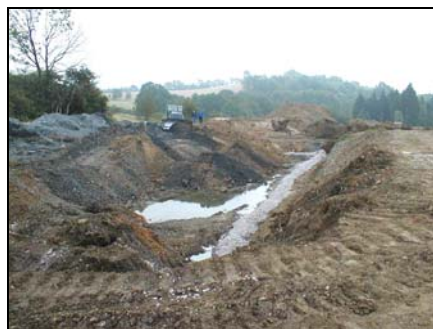
Filling the lagoon with inert material
