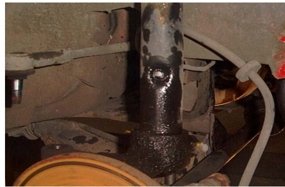
Drain of oil from the shock absorbers
